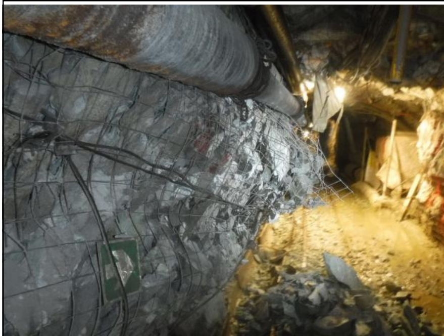
X-cut damaged (scaling sidewall)
