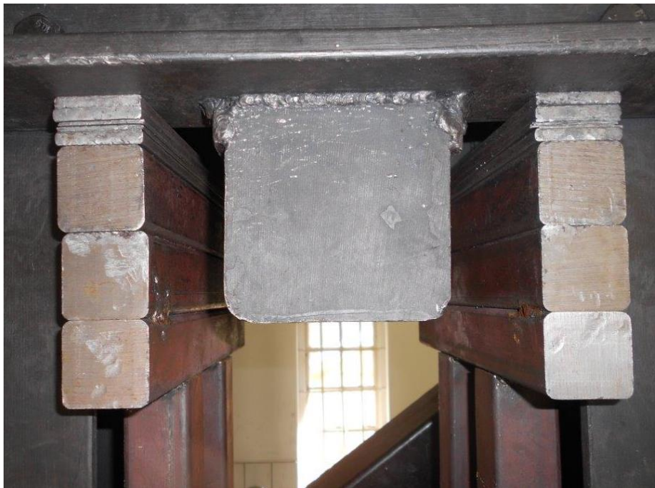
Figure 6. Assembly of vertical stand and shims abutting the top horizontal beam
