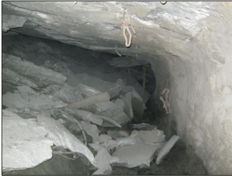
Figure 5: View along the ASG
