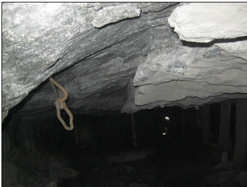
Figure 10: Fracture plane originating from stope face
