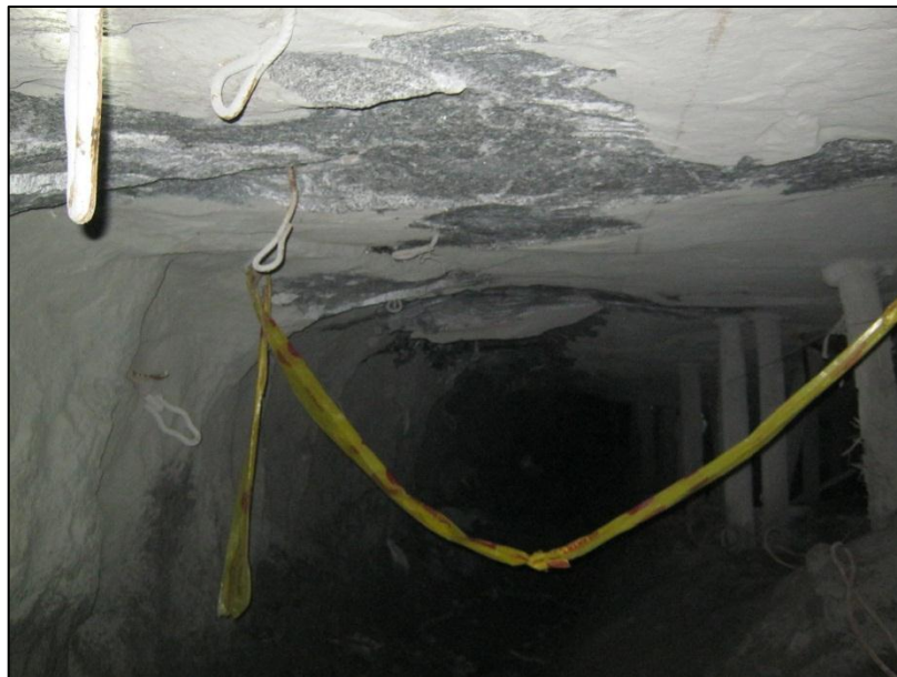
Figure 6: View along the ASG
