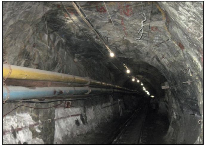
Figure 10: Dog earing on the top south corner of a crosscut.
