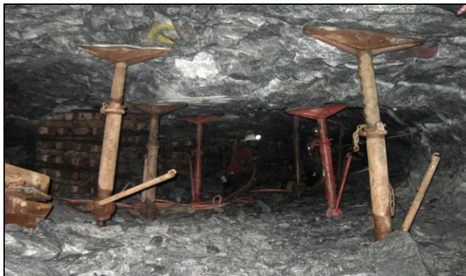
Figure 3: Two lines of temporary support provide a safe working environment between the permanent pack support and the face.
