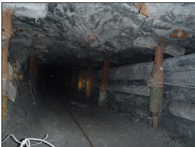
Figure 13: Blast barricades on front row of props
