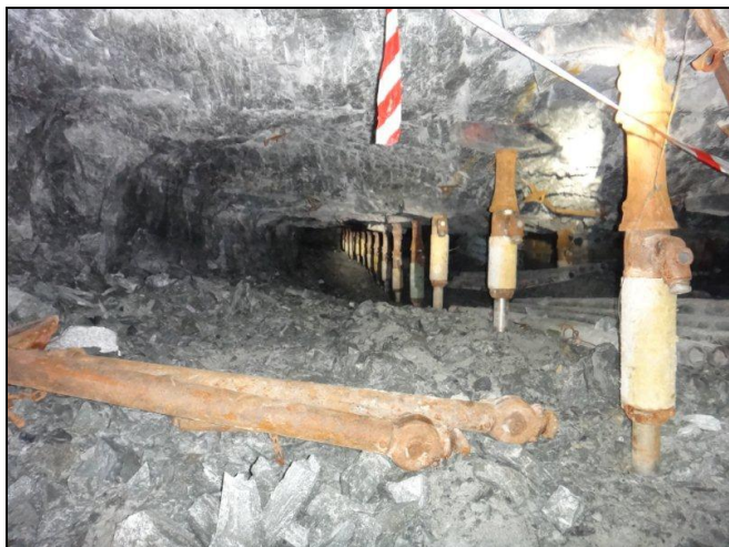
Figure 12: Two lines of hydraulic props, front row 1.5 m from face
