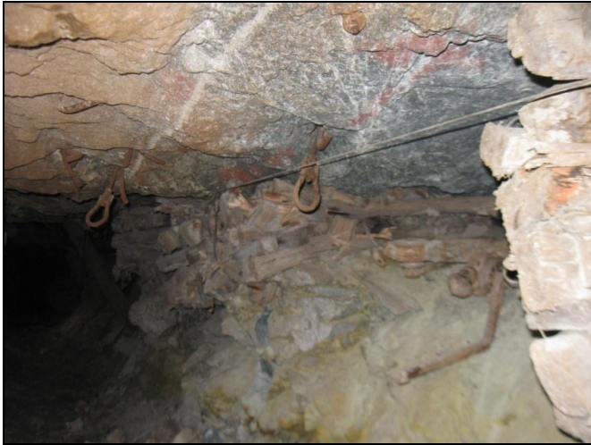
Figure 20: 60 cm of elastic closure on 120 cm high packs with no evidence of inelastic closure 45m behind a face.
