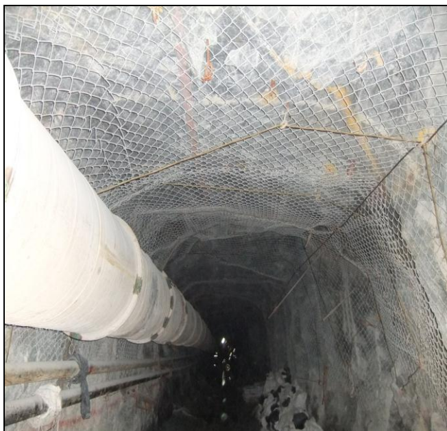
Figure 19: Mesh and temporary lacing used in tunnels.
