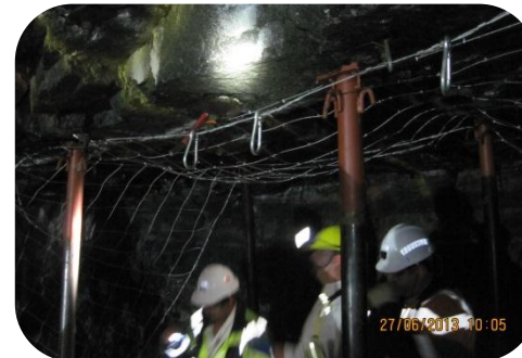
Completed installation of remotely installed hydraulic jacks with a safety net providing temporarily support access to affected area with safety net providing aerial coverage in the affected area
