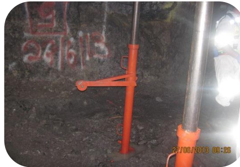
Guide bracket is then secured to the installed hydraulic jack
