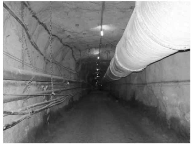
Figure 10 Showing fibrecrete and resin-grouted rebars in deep, fractured ground conditions
