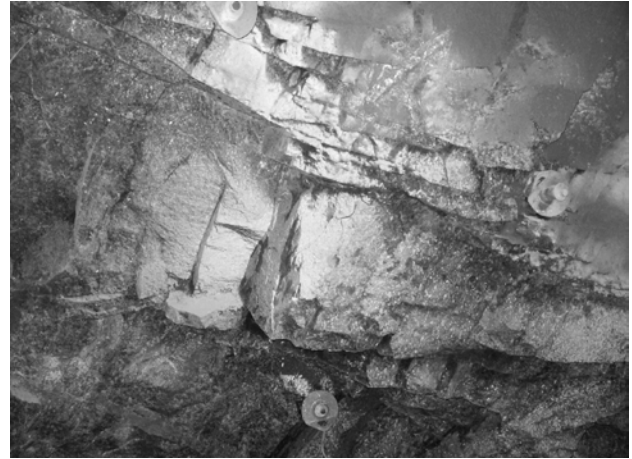
Figure 5 Typical "blocky ground" conditions as at No 20 shaft
