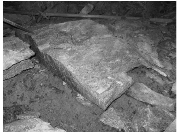
Figure 7 Thick "slab"-type stress-fractured block in noritic rock type at No 17 shaft
