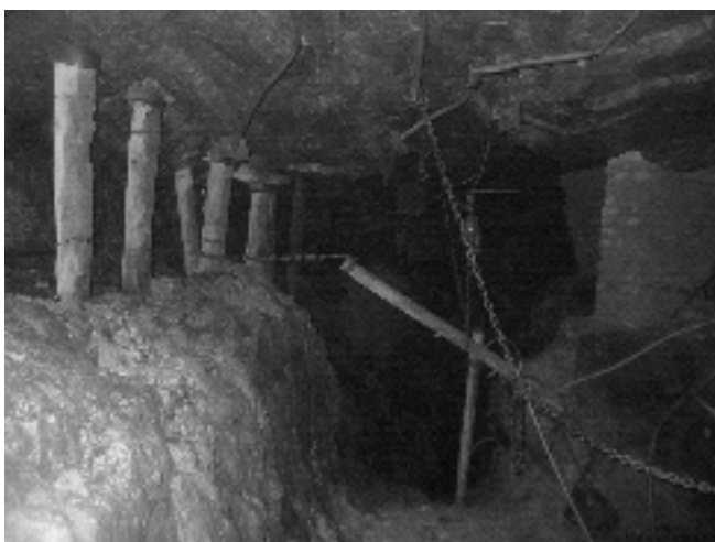
Figure 10. Photo of the exposed splitsets in the connecting gully during the ledging phase
