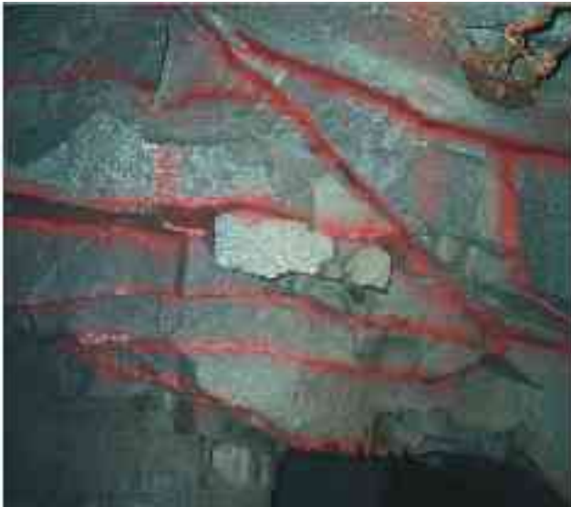
Photo 1: Condition of W1 gully hangingwall.
