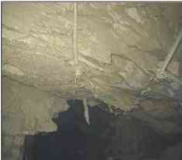
Photo 3: Condition of W1 gully hangingwall following application of TSL.
