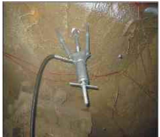
Photo 5: Pull tester used to determine in-situ bond strengths.
