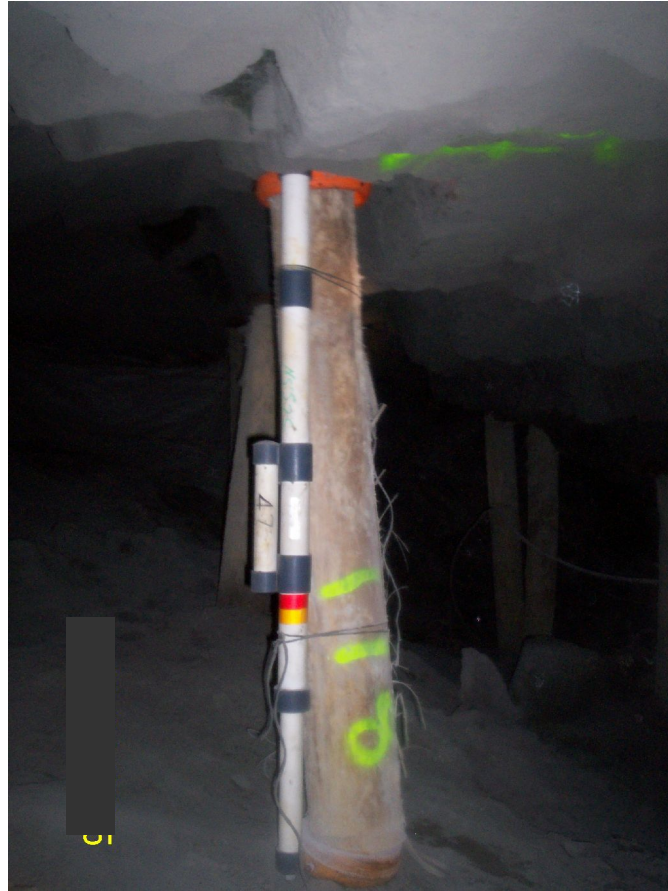
Figure 7. Closure and Load Loggers installed with a mine pole in a shallow platinum mine
