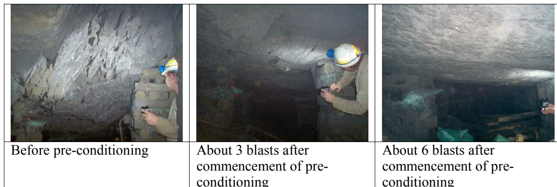
Figure 10: Illustrating the improvement in hangingwall conditions due to pre-conditioning and close supervision.
