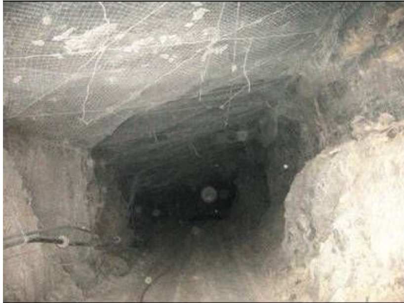
Figure 2. Mesh and lace used in parts of the access roadway
