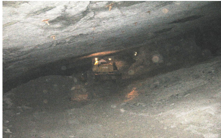
Figure 12. A dozer operating in a 12m wide roadway
