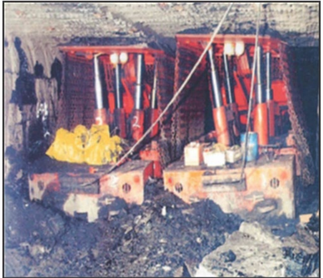
Figure 37: Mobile roof support units (Courtesy Fletcher et al.)
