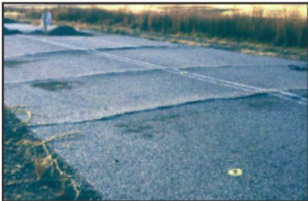
Figure 4: Compression humps
