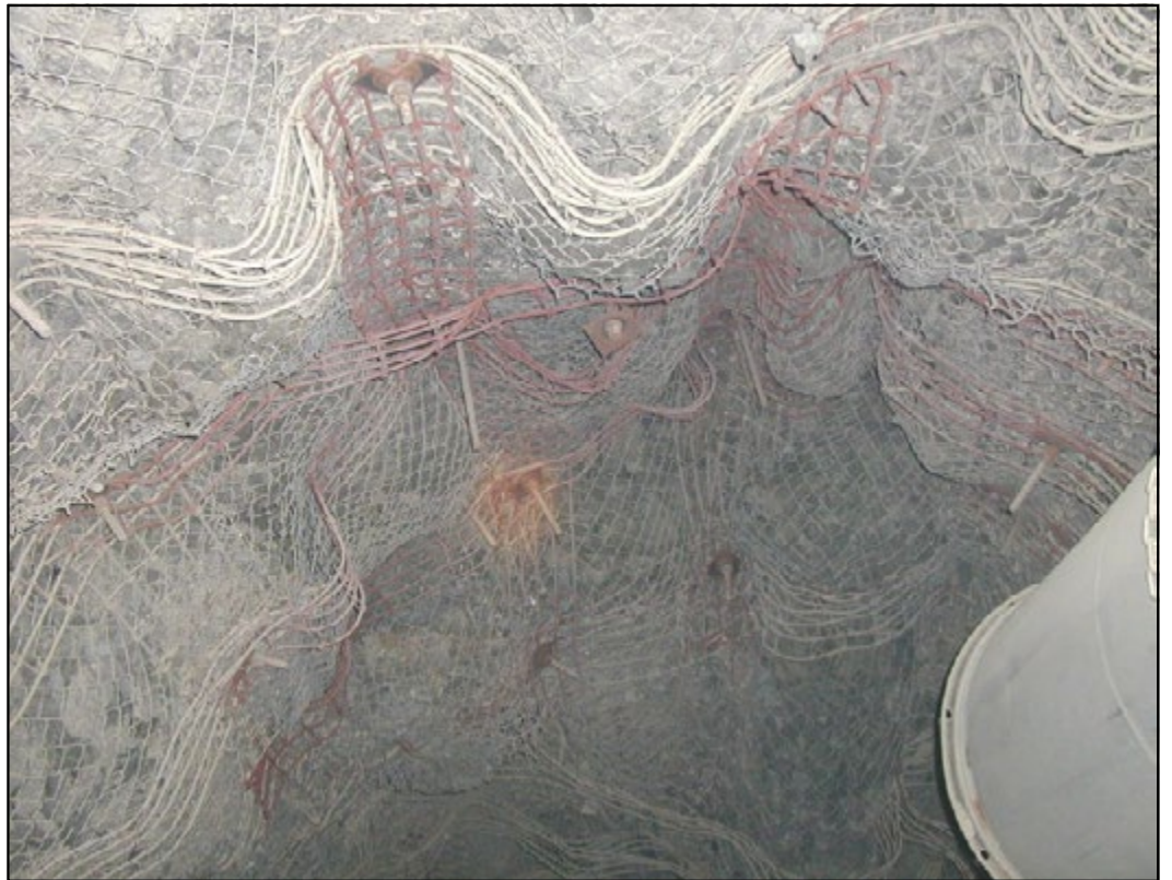
Figure 16: Mesh, anchors and Steel strapping in drawpoints (Courtesy of Petra Diamonds)
