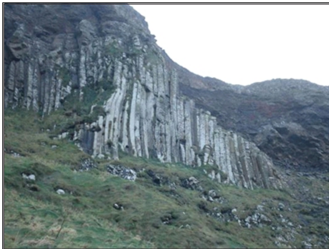
Figure 14: Steeply jointed rock in which toppling failure is highly likely
