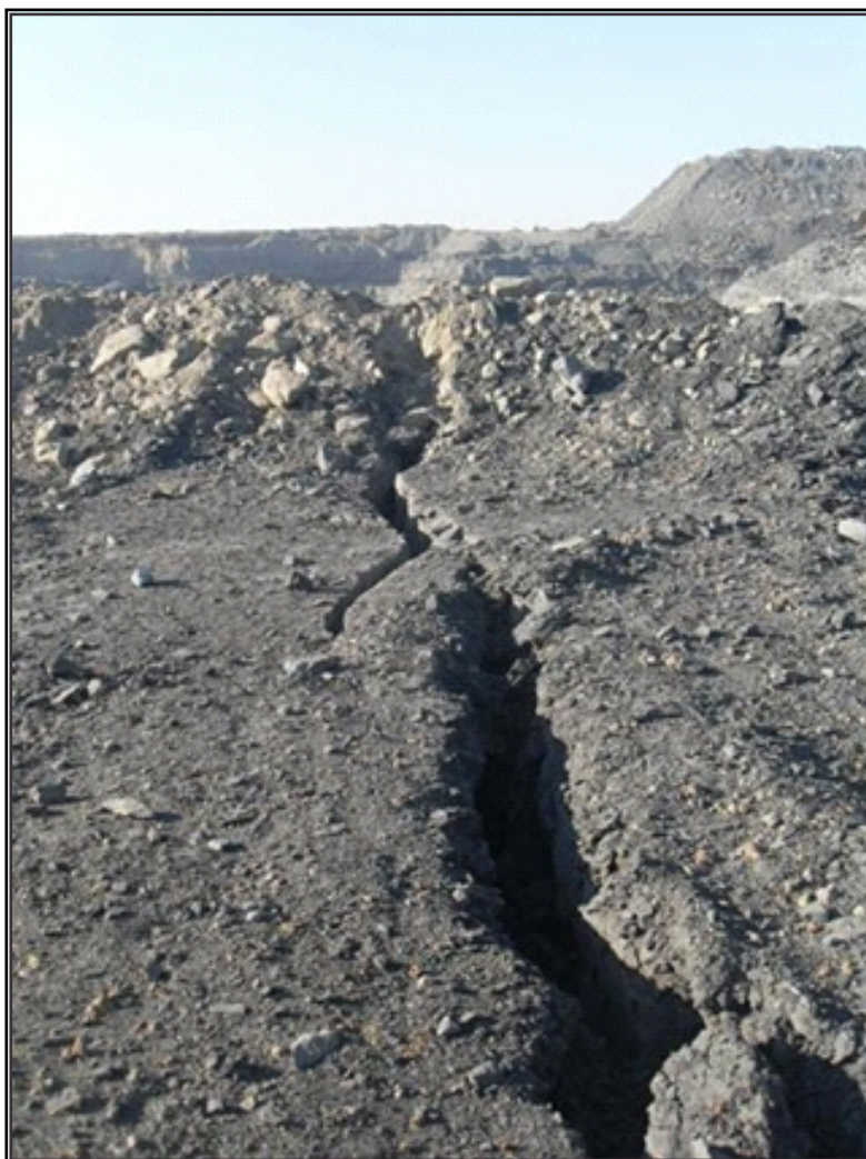
Figure 17: An example of a tension crack that has formed in hard material (Middindi, 2010) Link
