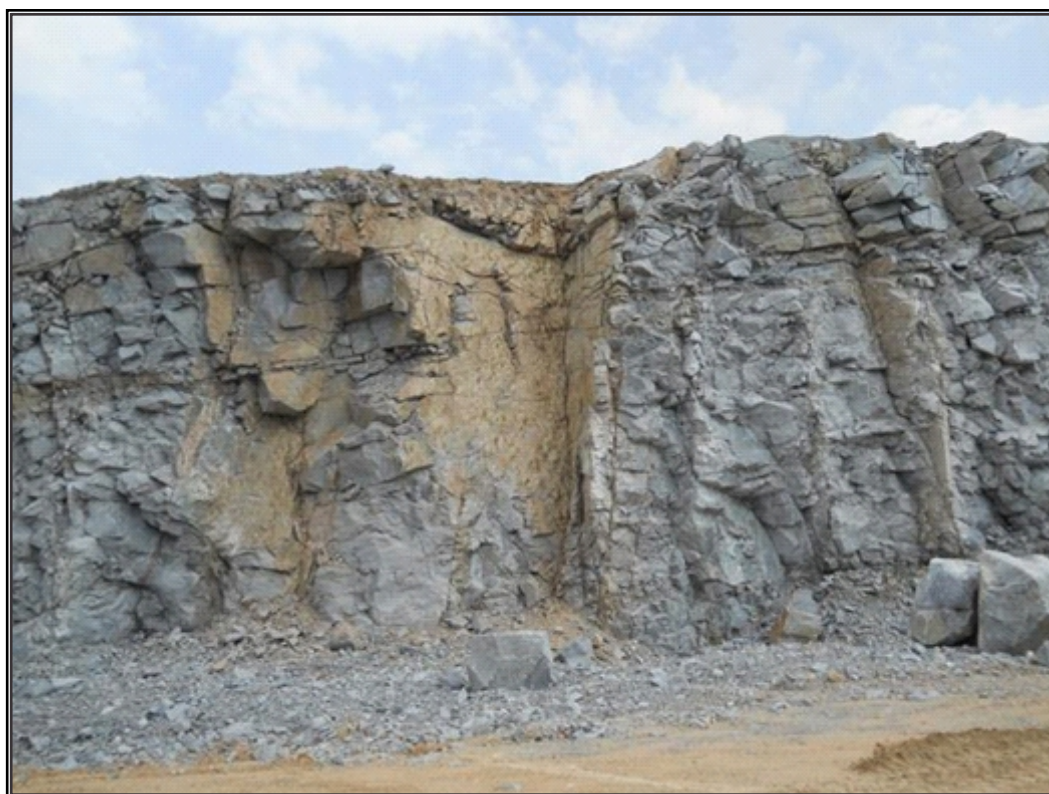
Figure 10: A steeper type of wedge failure (Middindi, 2010)
