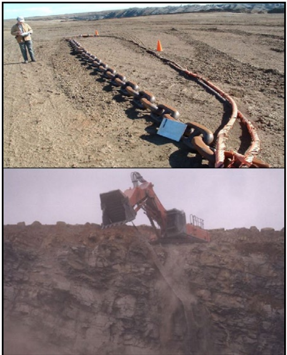
Figure 1: Making safe with chains
