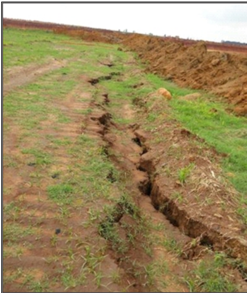
Figure 16 An example of tension cracks that have formed in soft material (Middindi, 2010)
