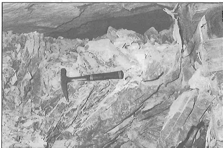
Figure 8.3.4 Rock ejected from the footwall and face between F and G (see Figure 8.3.1) into the space between the original face position and the first dip line of packs. The photograph is taken looking updip with the face to the left. Note the intact hangingwall.
