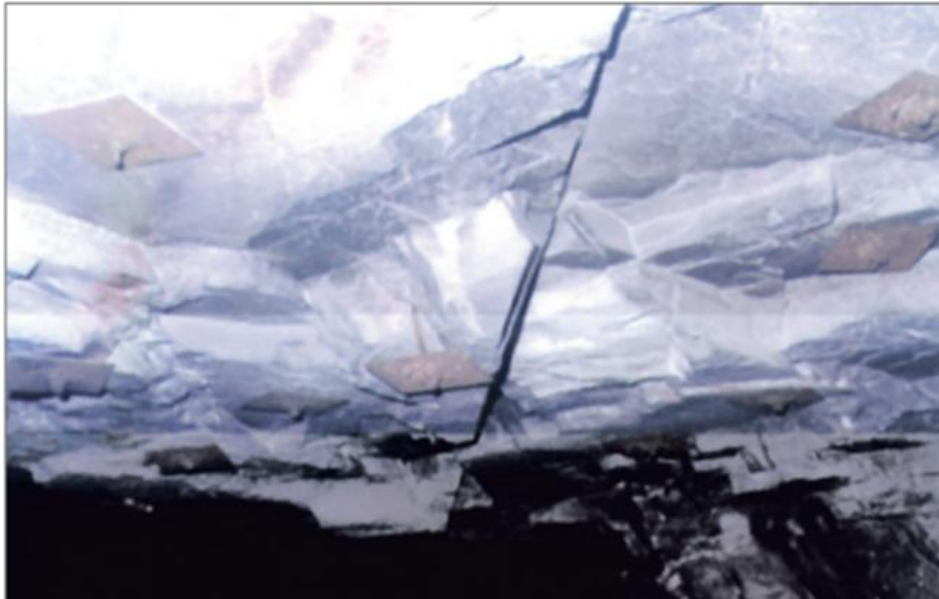
Figure 1: Immediate sandstone roof in an incline development at approximately 180 m below surface.
