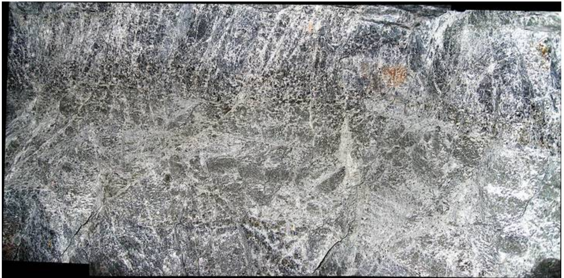
Figure 34: Fractures in the sidewall of a CLR stope at TauTona
