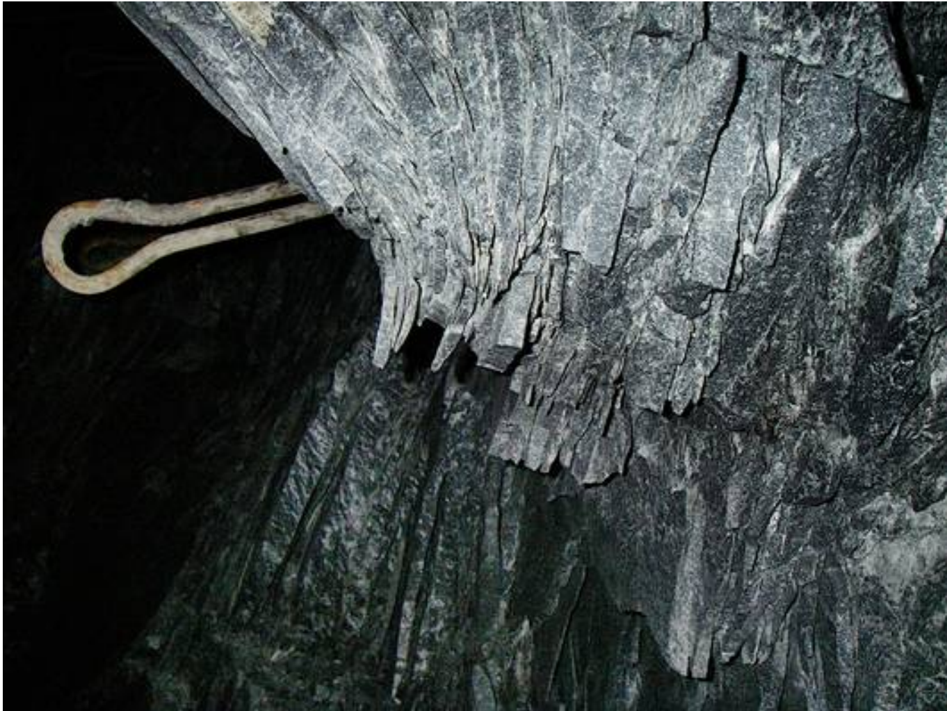
Figure 46: Curving extension fractures - we see it all the time ...
