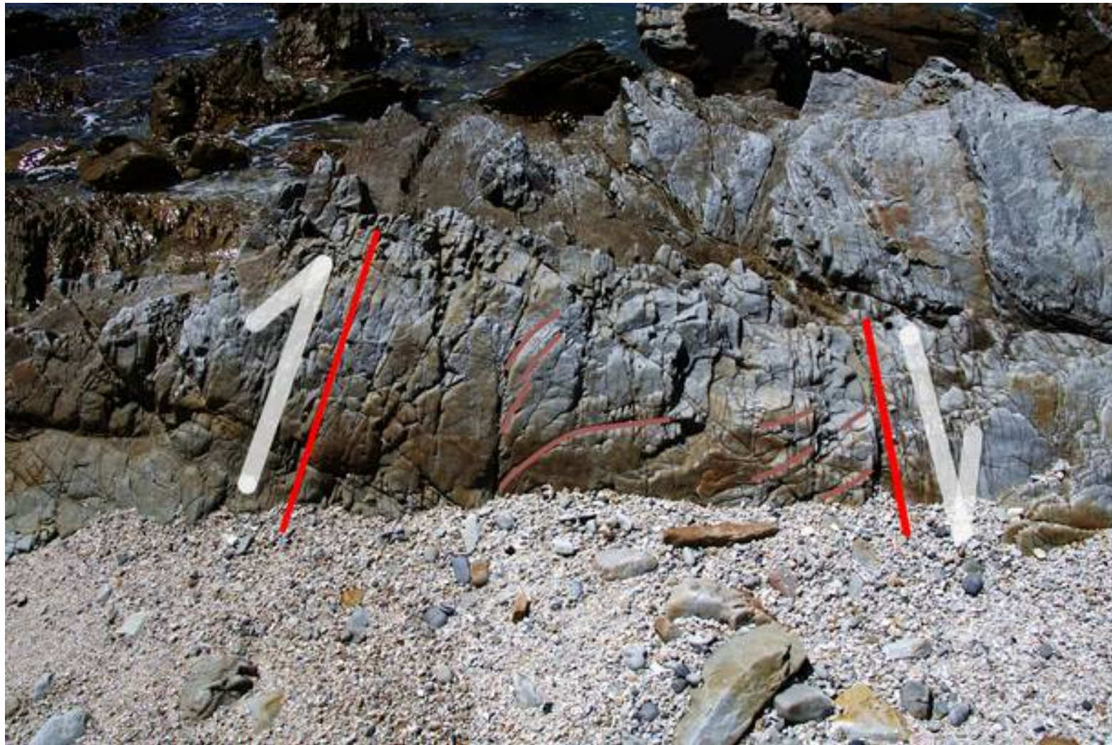
Figure 47: Curving extension fractures in a brittle shear zone near Kleinbaai
