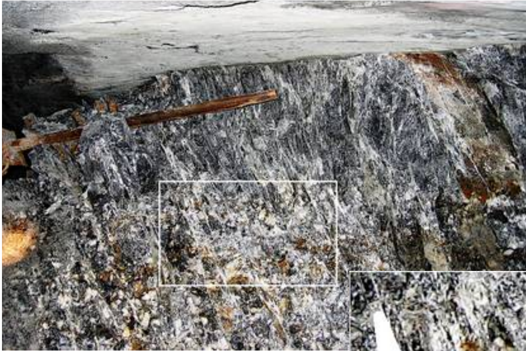
Figure 12: Extension fractures ahead of a VCR stope at Tau Lekoa showing shear displacement when the face got close.
