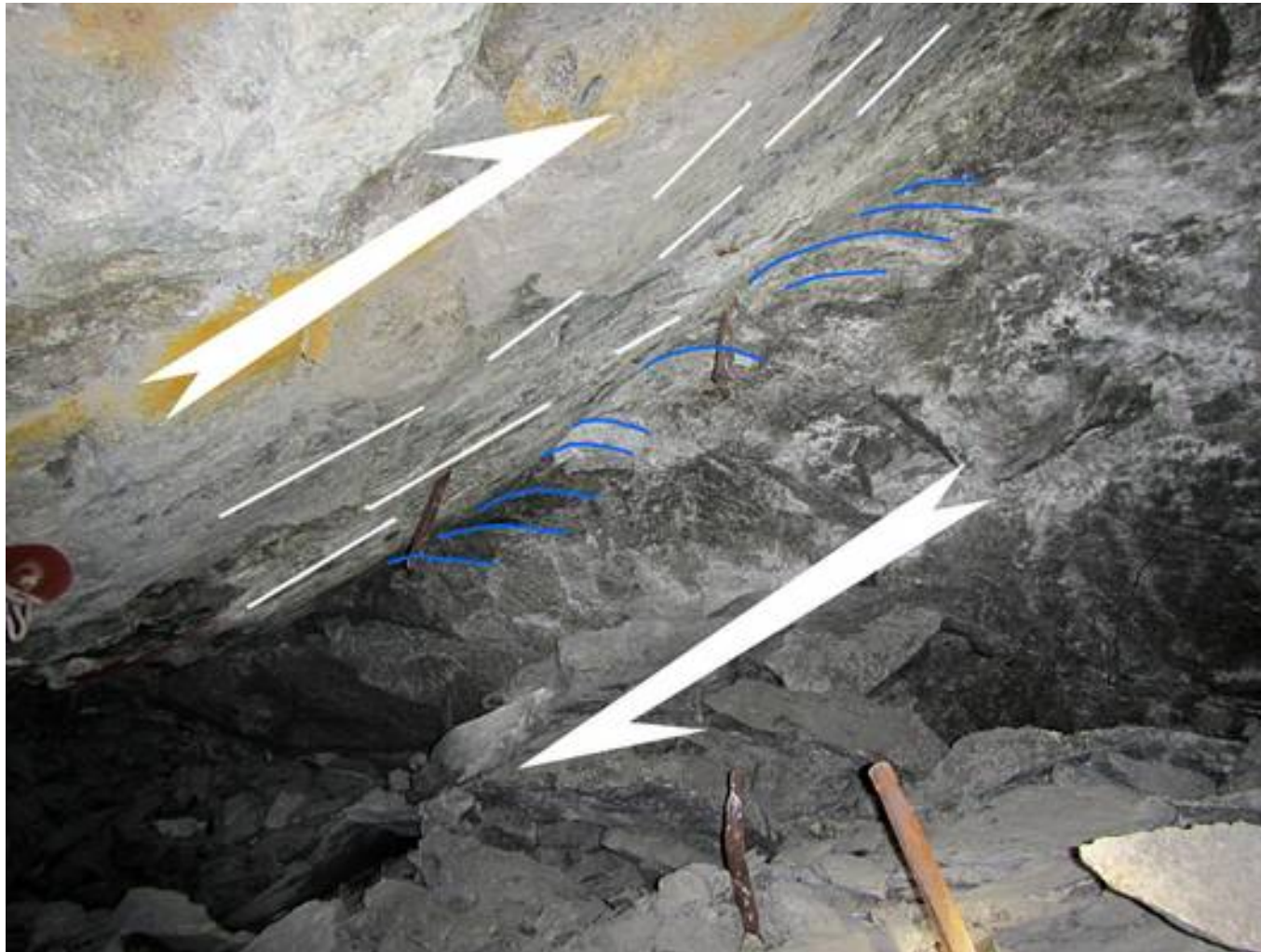
Figure 54: Rockburst mechanism at Siphu indicates principle stress is NS - again
