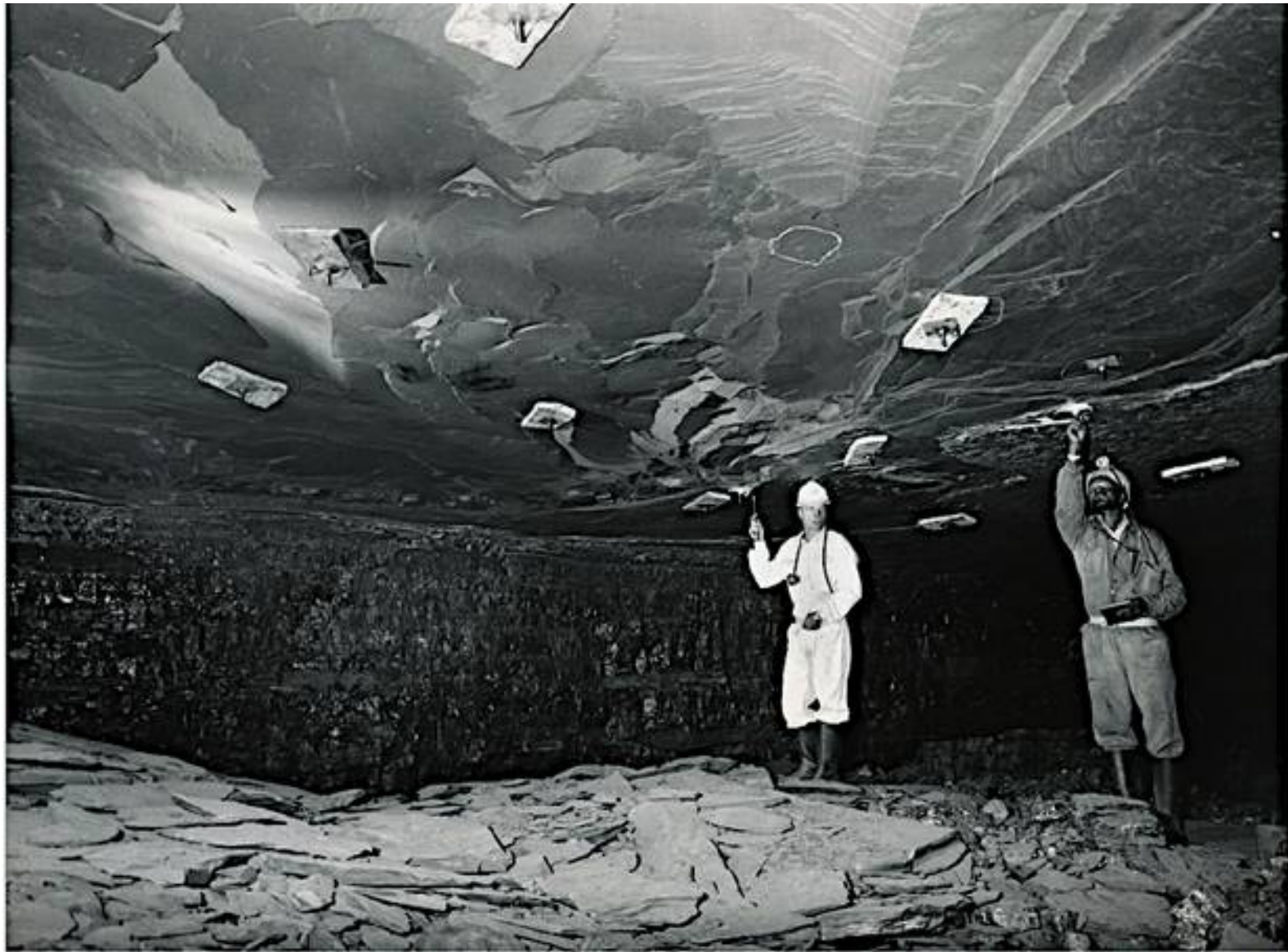
Figure 14: Buckling of the roof in a shallow coal mine (Ortlepp, 1997)..
