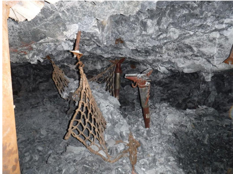
Damage in a stope face
