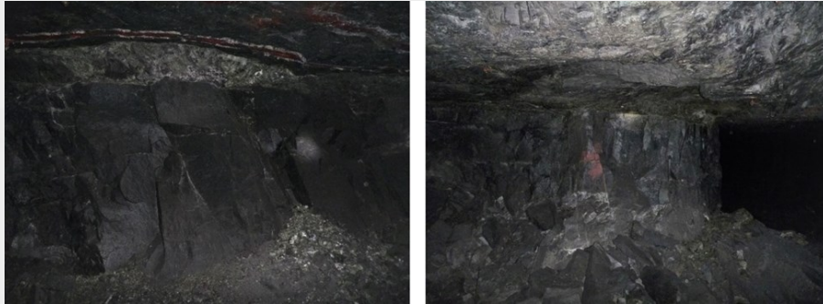
Figure 3: Pillar-forming material at Everest Mine which includes an altered layer along the top of the pillar contributing to the pillar instabilities experienced at the mine.
