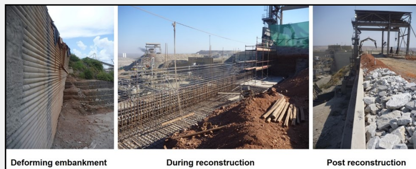
Figure 4: Reconstruction of crusher retaining embankment.
