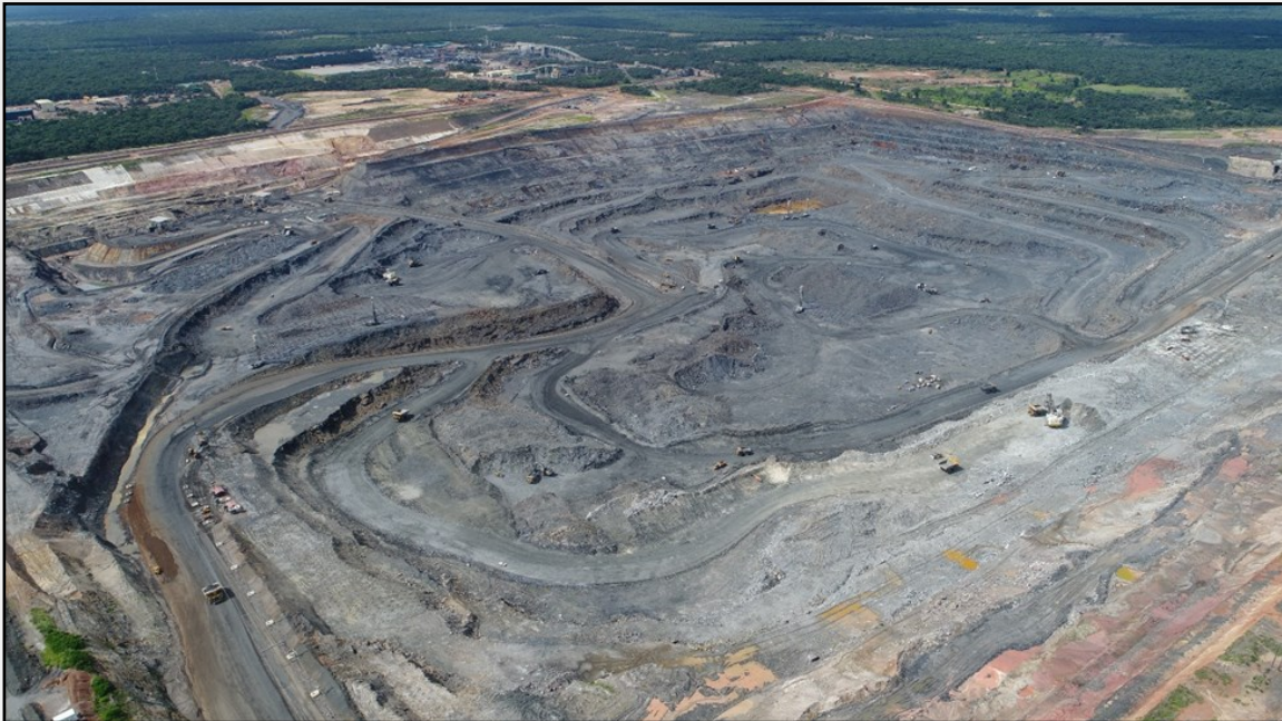
Aerial photograph of Sentinel Mine.
