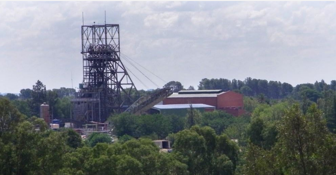
Loraine mine shaft
