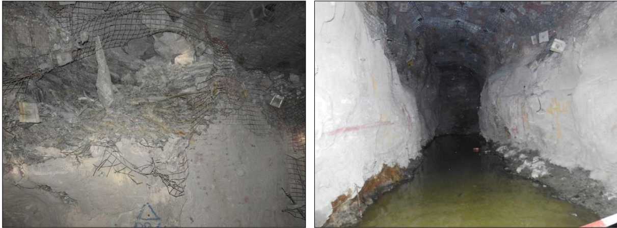
Figure 4. The photograph on the left shows sidewall mesh failure above the shotcrete following a ML 1.7 seismic event. The photograph on the right shows the ability of the shotcrete applied over the mesh to contain any potential sidewall damage following a ML 0.8 seismic event (right hand sidewall)
