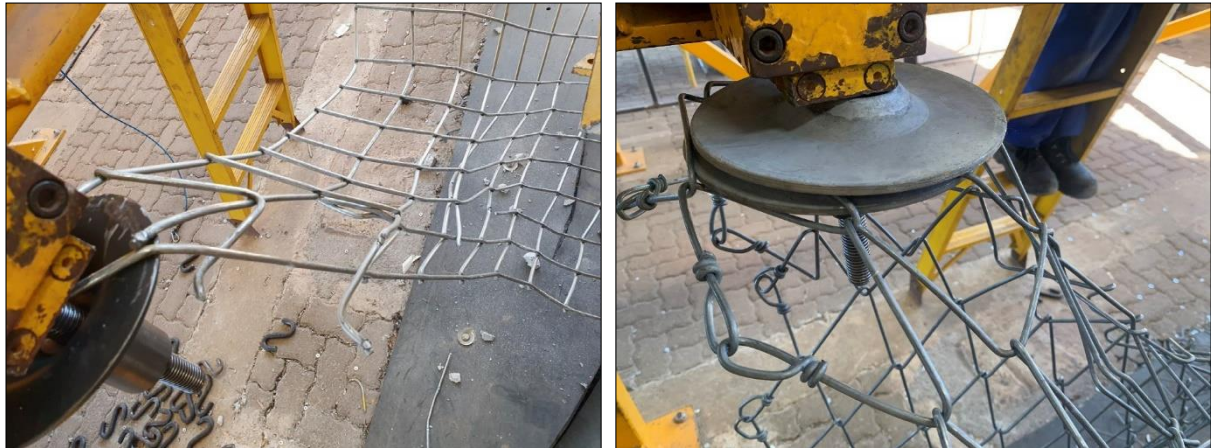
Figure 12. The photograph on the left indicates the premature failure of mesh strands as loading takes place against the rockbolt rather than the faceplate (single faceplate set up). The photograph on the right indicates good interaction between the faceplate and mesh (double faceplate set up). The transversal loading was limited and the performance of the mesh was reliant on numerous strands interacting with the faceplate
