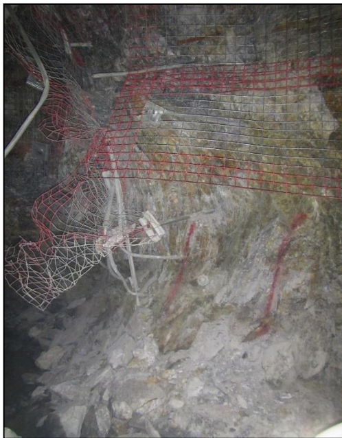
Figure 3. The damage resulted from a ML 2.2 seismic event. Notice the inability of the system (rockbolt and mesh) to absorb the impact of the ejection. The stiff mesh folds around the bolt which did not engage the yielding mechanism
