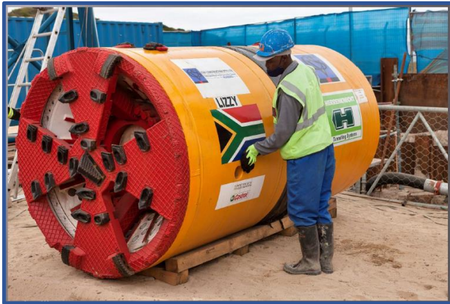
Microtunnelling in Cape Town
