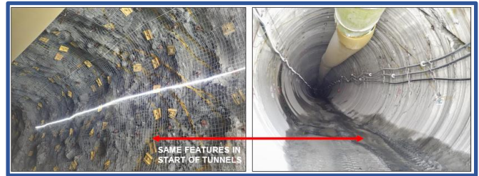
Drill and Blast tunnel viz. with Mobile Tunnel Bored tunnel
