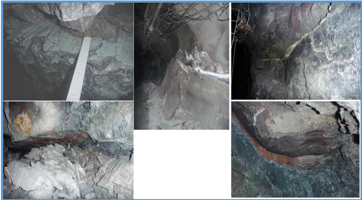
Figure 3: Yielding mechanisms of the pillars (Sliding along shear planes or punching into footwall)
