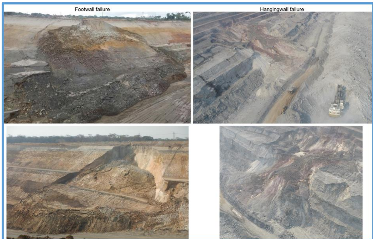
Figure 8: Multi-bench failure in weathered material
